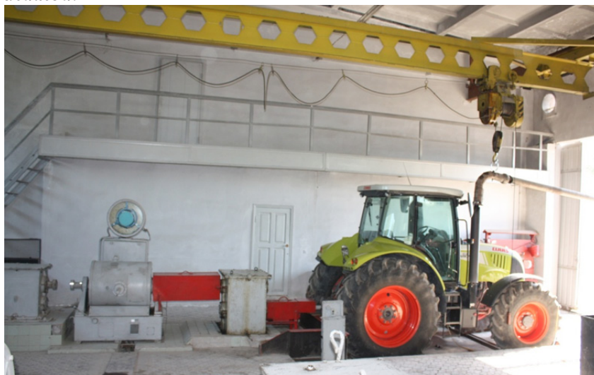
Figure 1. Electro-brake stand GPF-5–17N with weighing device “Rapido” in working condition when testing the tractor engine
