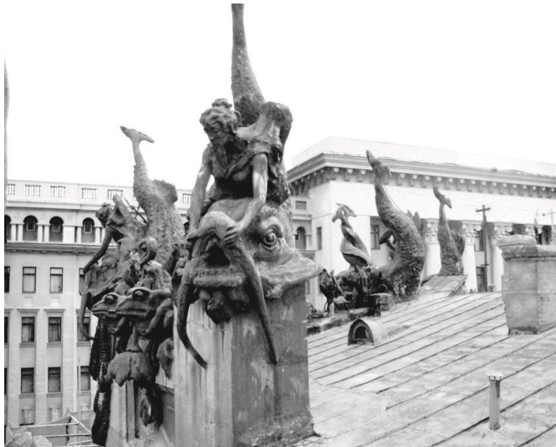
Figure 1. Fragments of the sculpture destruction on the “chimera house” roof before restoration 2001
