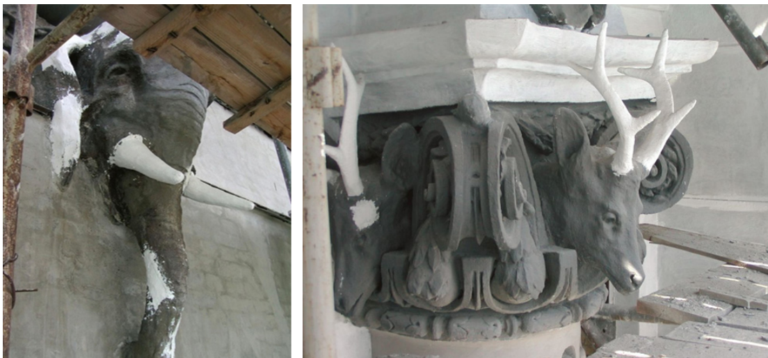
Figure 2–3. Restoration of stucco figures on the “chimera house” facade in 2002
