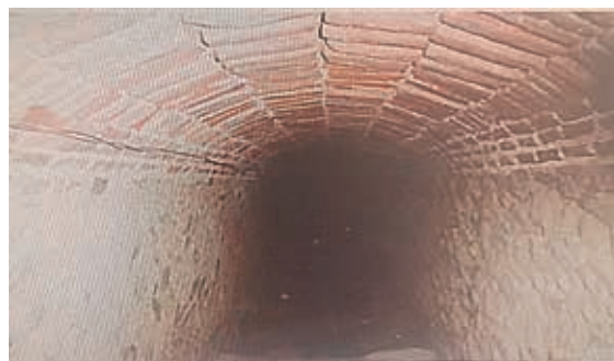
Figure 2. The entrance of “Girhpille” made of for descent into the well at Ordubad Azerbaijan [4]
