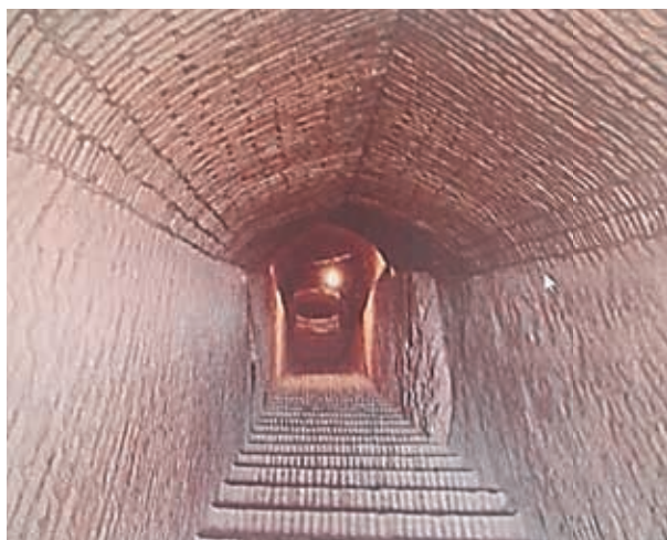
Figure 1. The entrance of "Girhpille" made of for descent into the well kyariz at Yazd, Iran [4]
