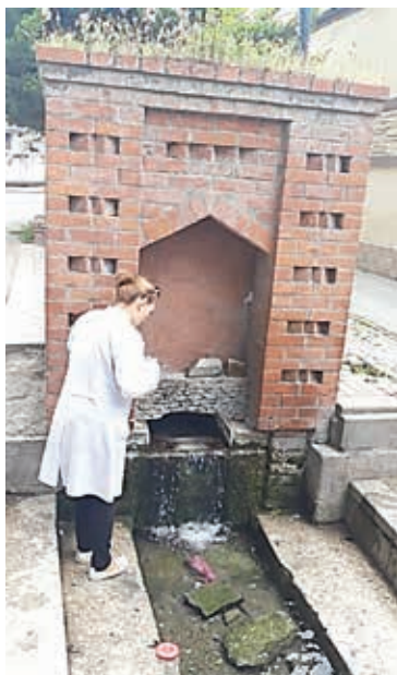
Figure 3. The pool and drenagge chanel at exit kyariz in Ordubad [4]
