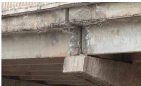
Photo 4. Corrosion of the crossbeam concrete and a network of cracks on its surface
