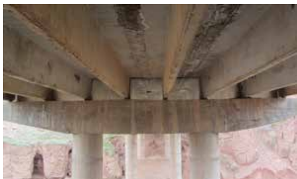
Photo 3. Through-crack in the middle of the outer beam of the span, with a crack width of up to 5 mm
