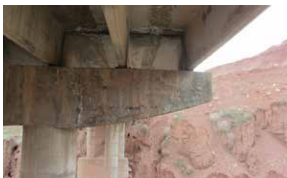
Photo 6. Damage to the lower part of the beam rib
