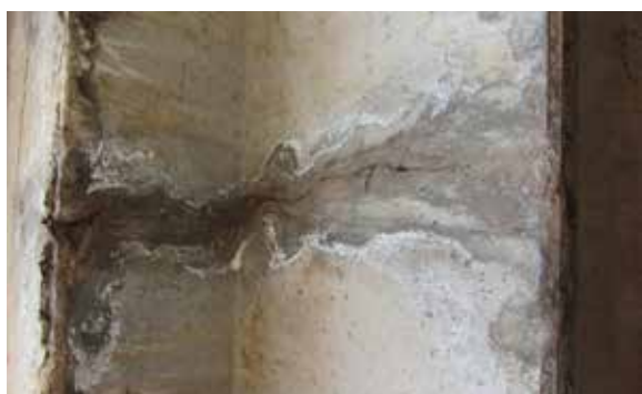
Photo 5. Scouring of the bridge foundation
