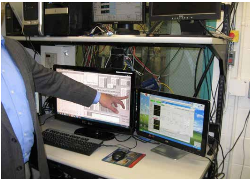
Figure 2. Example of an integrated startup workstation
