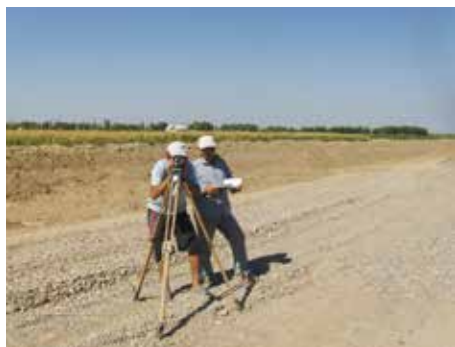
Fig. 2. Geodetic layout work
