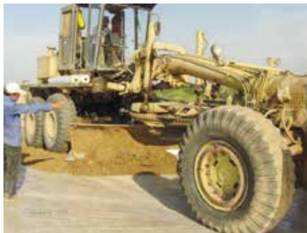
Fig.8. Backfill with the second layer
