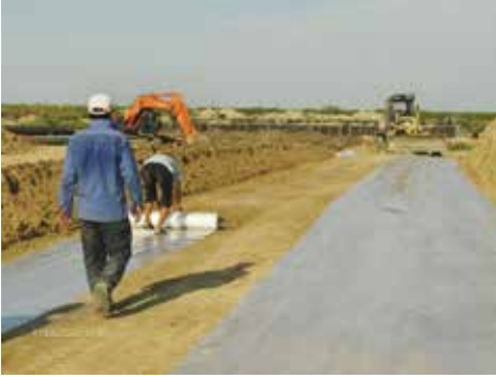
Fig. 3. Rollout with tension
