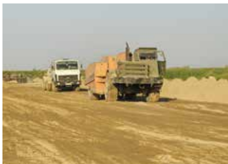
Fig.7. Soil compaction by a road-roller on a pneumatic run
