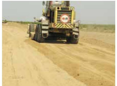
Fig. 6. Leveling with a motor grader
