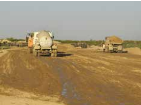
Fig.5. Landfilling by the «push away» method
