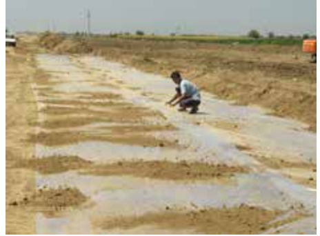
Fig.4. Rollout with overlapping
